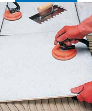
Laying large size tiles
