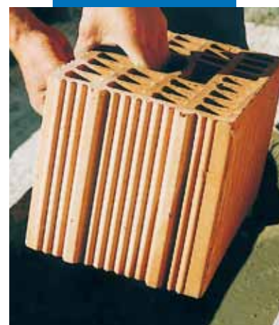
Dipping a concrete block in Adesilex P4
