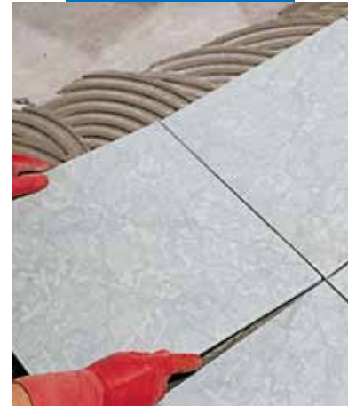
Laying porcelain tiles
