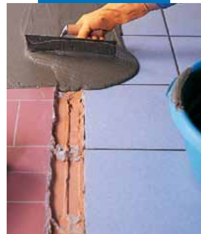
Smoothing existing flooring with Adesilex P4
